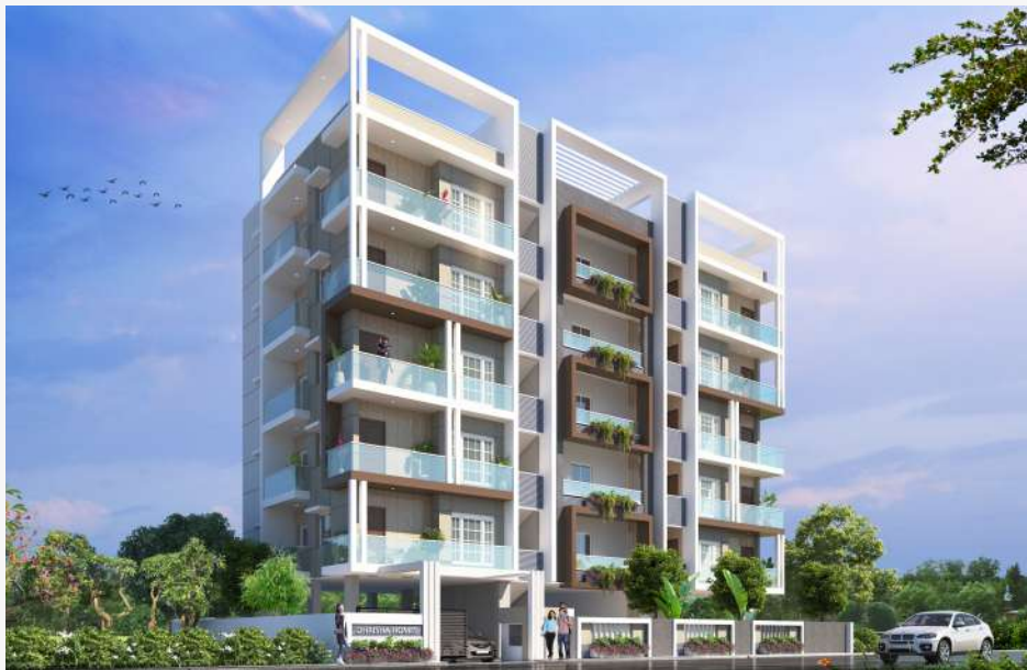
SREE DHRISHA HOMES MIYAPUR
